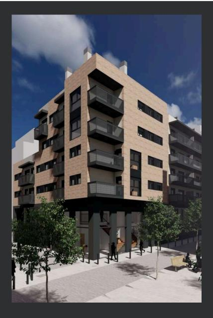
The building is designed in a rectangular shape, bordered by Corsega and Navas de Tolosa Streets. The development includes a community parking garage with storage units, spread across 2 basement levels, occupying the entire plot. On the ground floor, there are residences with direct access from the street, as well as 2 commercial premises located at the building's corner, the entrance lobbies to the homes, and access to the parking garage.
